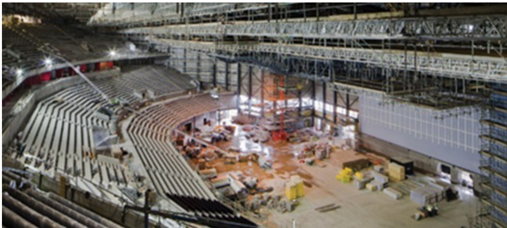
Figure 9.4: Actual building structure of the high profile cultural facility
